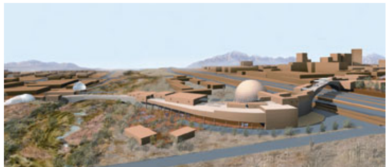
The proposed University of Arizona Science and Entertainment Center, spanning the I-10 Freeway in downtown Tucson, will become one of the most visible icons of the massive downtown redevelopment program.
